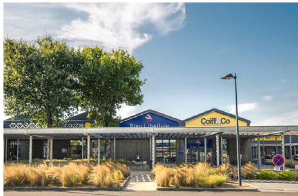
La Colleraye - Savenay (Hérault) - Centre commercial
